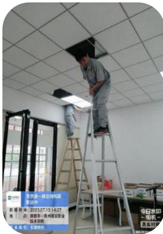
思贤楼一楼空调线铺设
